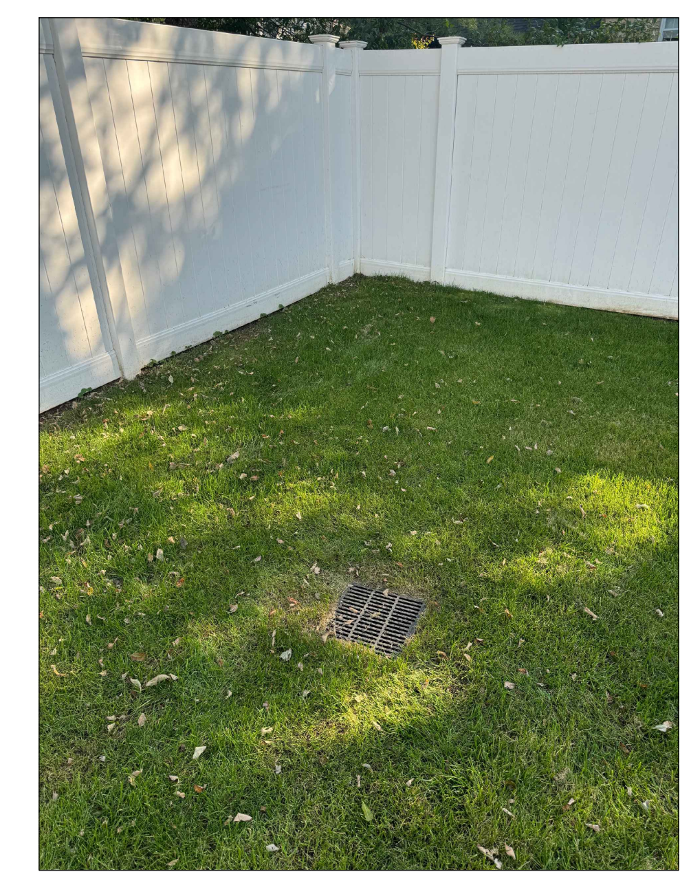
EXISTING PHOTO OF DRYWELL GRATE AT GRADE SCALE: NOT TO SCALE
